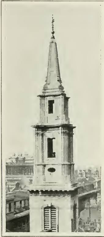
ST. VEDAST, FOSTER LANE, CITY OF LONDON.
